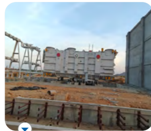
Transmission system in Raigarh II (BOOT)
