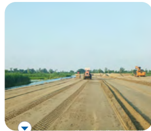
Kasganj Bypass (HAM)
